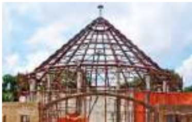
Raised part of the structure
