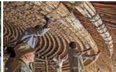
Decorative ceiling structure (Wamara tombs)
