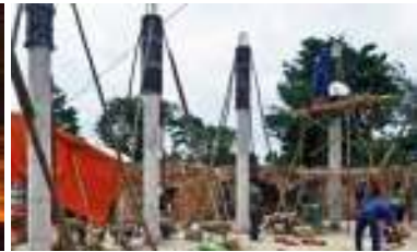
Construction of concrete poles
